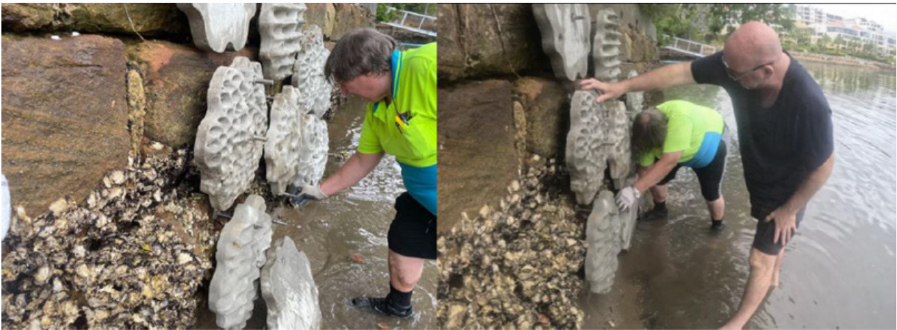
Images 24 & 25 - Installation of the Living Seawall panels
