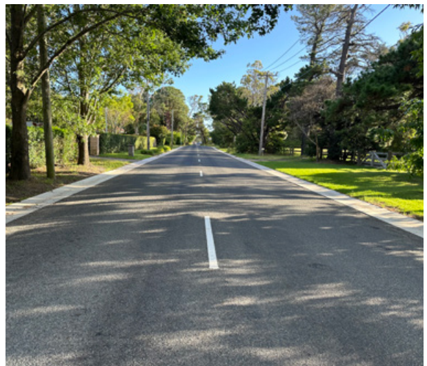
Cobah Road newest section of road. Image Source: Martin Pluss
