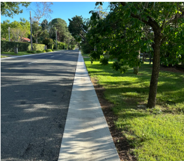
Cobah Road new style of gutter. Image Source: Martin Pluss
