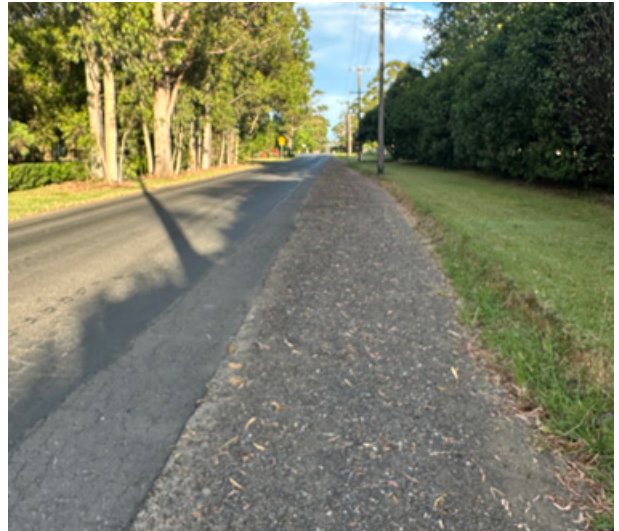
Cobah Road Gravel Verge. Image Source: Martin Pluss
