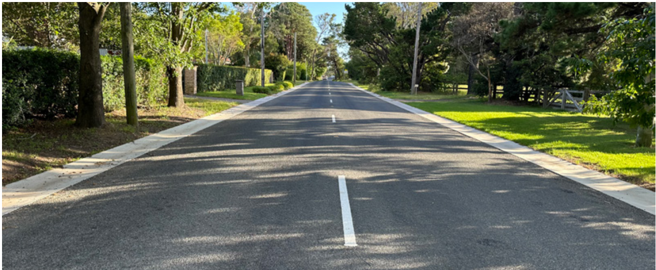
Cobah Road newest section of road. Image Source: Martin Pluss
