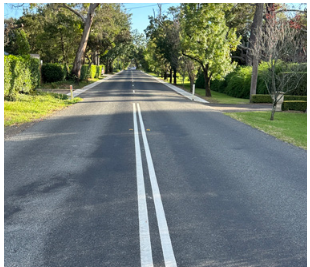
Cobah Road transition to new guttering. Image Source: Martin Pluss
