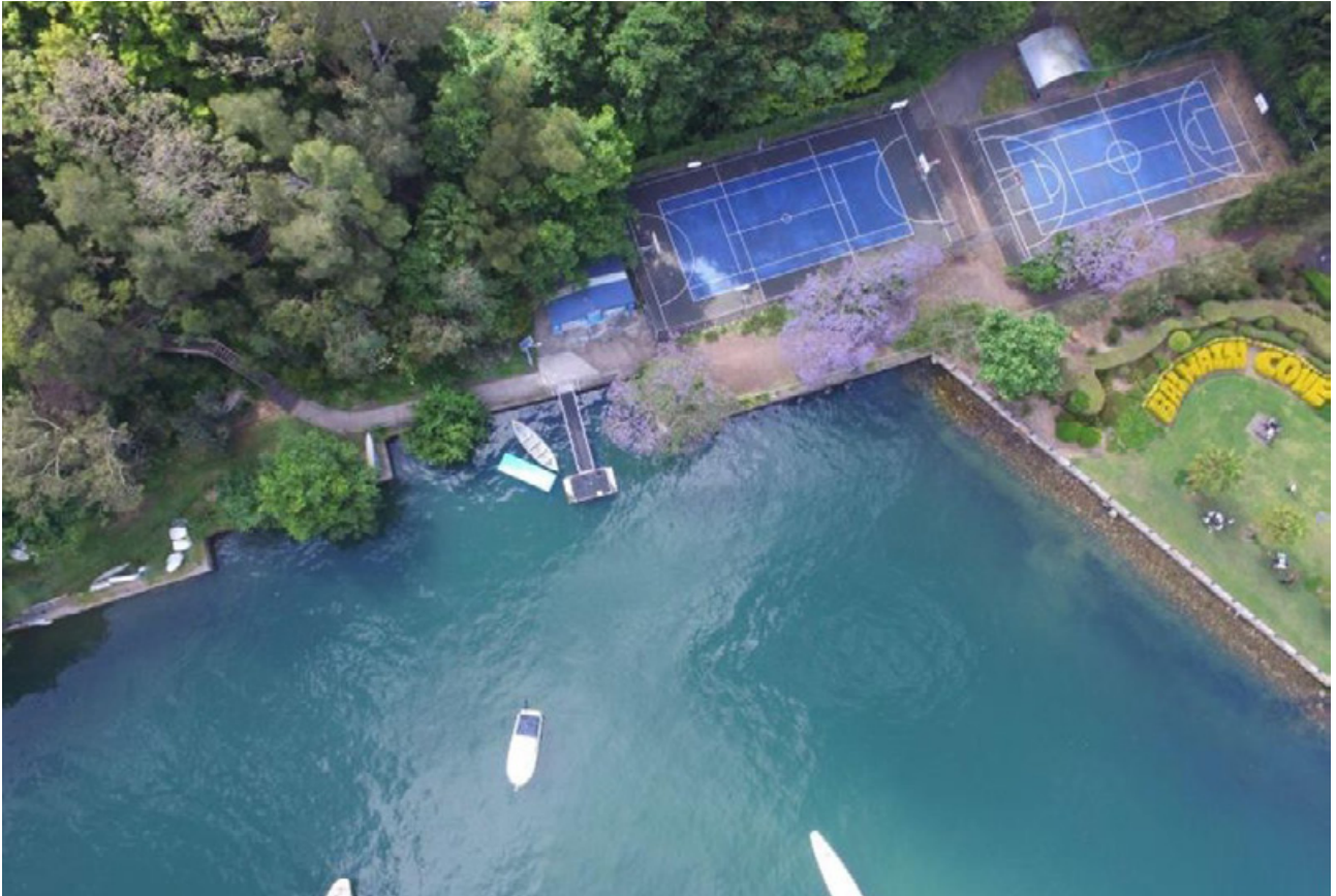
Image 1 - Aerial picture of SSCBC Foreshore
