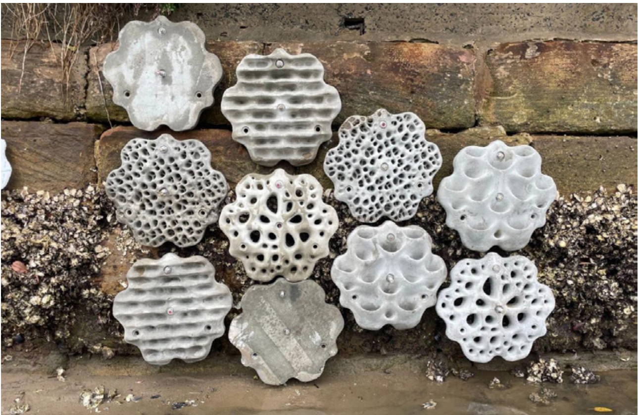
Image 26 - The Living Seawall panels installed
